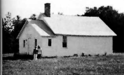
Perreault Station School
